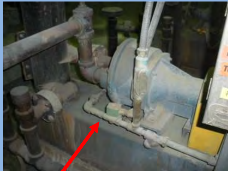
With Solenoid & Orifice <5gpm, and flow stops when pump stops.
